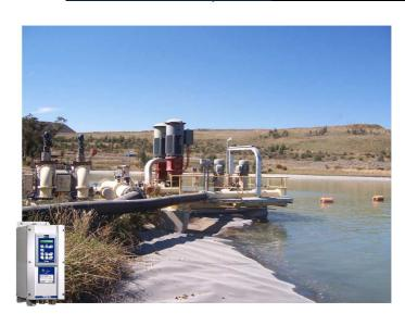
The TECO F33, 2.0 AC drive is specially developed for regulating flow and pressure. It continuously adapts motor speed to the level required, minimizing energy consumption and wear. A unique monitoring functionality protects your process from damage and unplanned downtime. Typical applications are pumps, fans, compressors and blowers.
